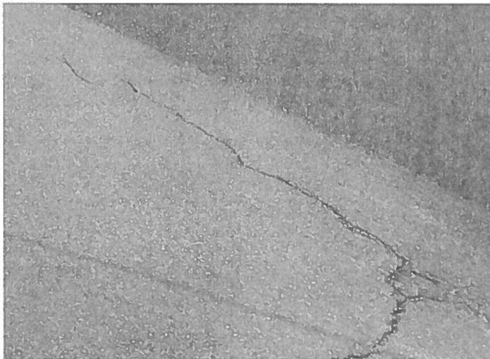
Figure 2: Medium cracking
