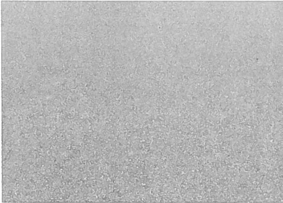
Figure 5: No defects, excellent condition
